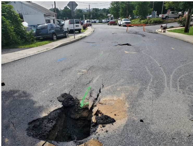
Figure 4.3.6-4: A small sinkhole opened up on Susquehanna Avenue in East Pennsboro Township due to flash flooding in 2021 (Photograph courtesy of East Pennsboro Township, 2024).
