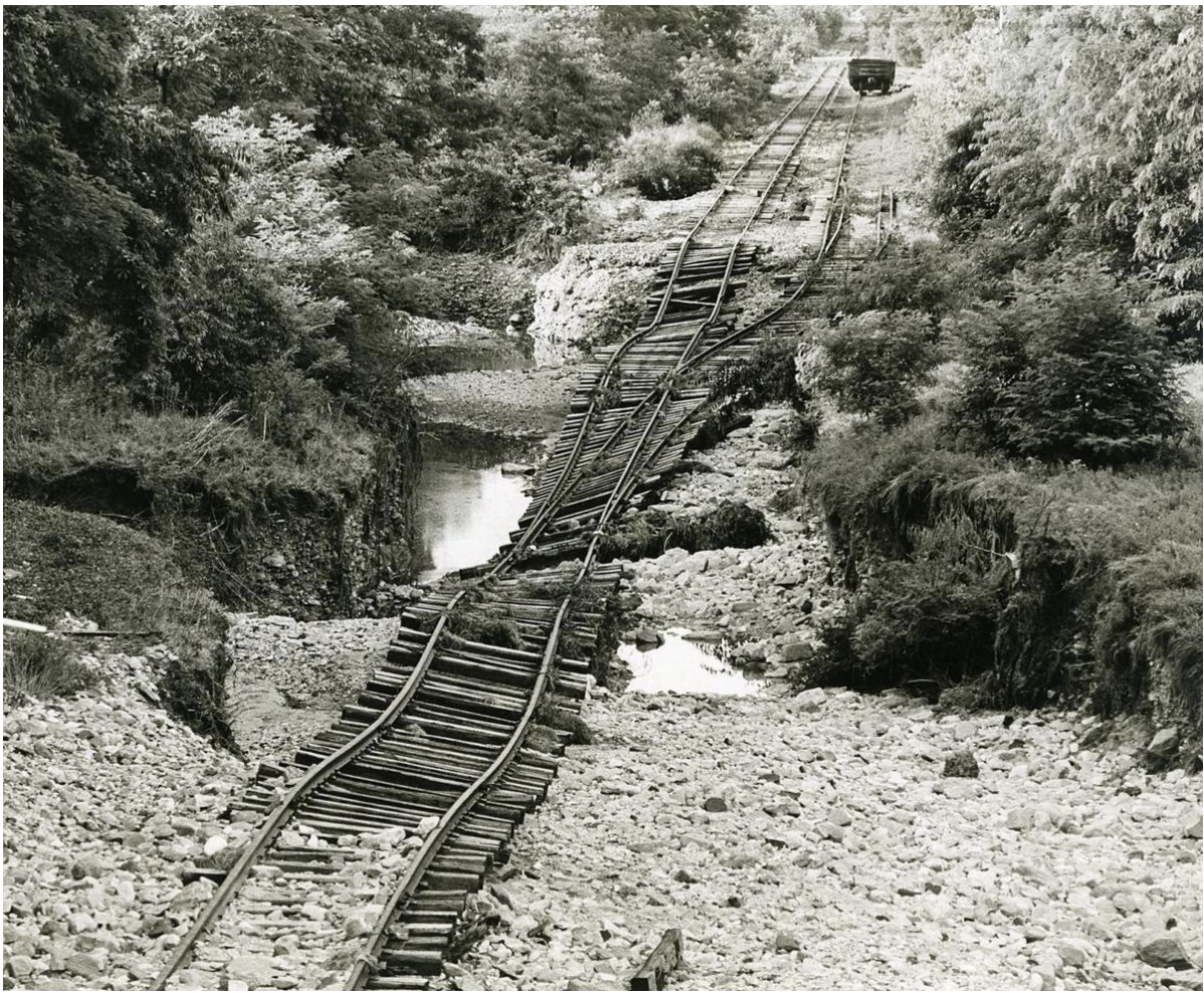
Figure 4.3.4-2: Flood damage to the Reading G&H Branch at Carlisle Junction (Cumberland County, PA), due to Hurricane Agnes (Photograph courtesy of Michael Bupp/ The Sentinel , courtesy of the Cumberland County Historical Society, 2018).
