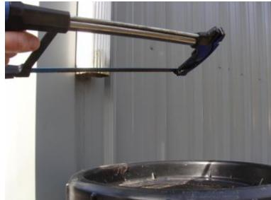
Cut your existing downspout about 6" to 12" above the top of the barrel
