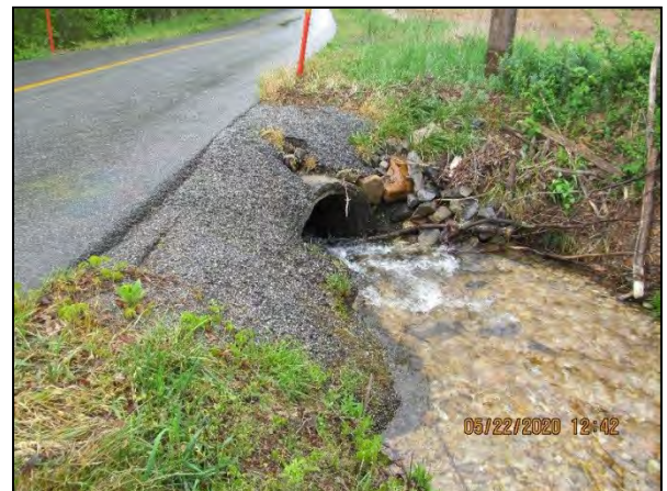
Furnace Hollow Road Culvert to be replaced in 2021.
