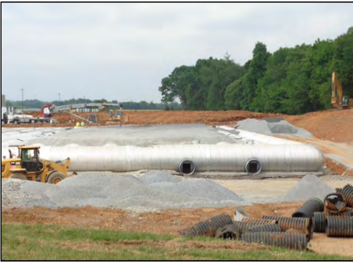
Underground Stormwater Best Management Practices installed for Post Construction Stormwater Management
