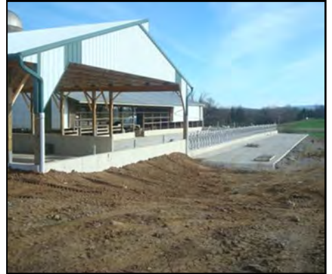
Roofed Waste Storage Area and Heavy Use Area Protection.
