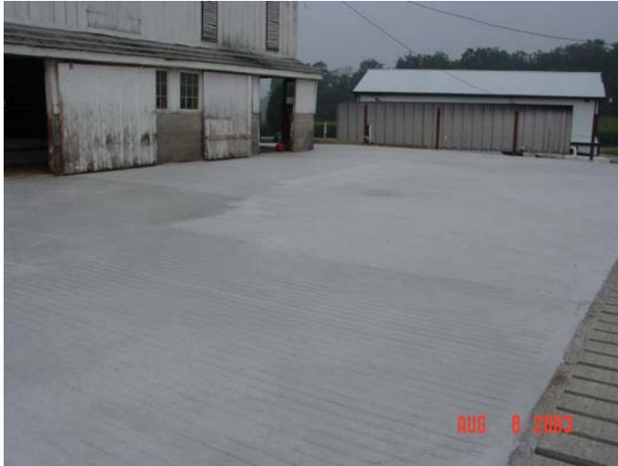
Heavy use area concreted to reduce runoff
