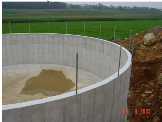
Manure storage structure in near completion
